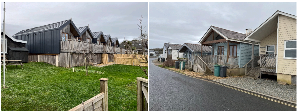
Fig. 7. Examples of structural accommodation measures on the Isle of Wight, south coast of England. A void area is located below finished floor levels. Over half the buildings in this floodplain have been rebuilt and raised from grade in the last 20 years.
