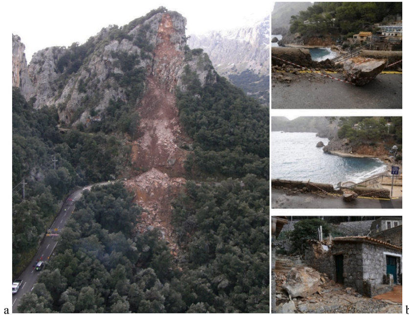
Fig. A1. a) Gorg Blau rockfall (Tramuntana range) occurred at the end of 2008 after heavy rains and low temperatures. The main road of the region (Ma-10) was blocked during almost 3.5 months. b- Rockfalls at Sa Calobra during the rainy event in 2019.
