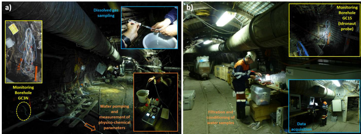
Fig. 2. (a) View of the CARBOLAB gallery with insets focusing on the monitoring technics used; (b) View of a lateral gallery where the material is stored with details on the installations.
