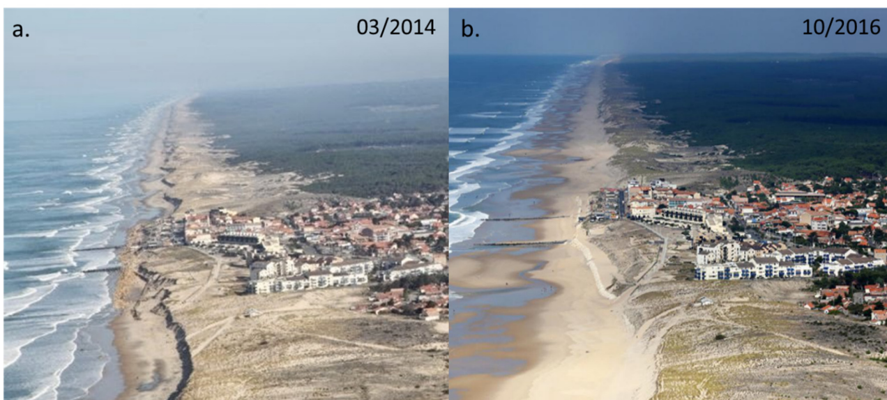
Figure 13. Aerial photographs of Lacanau from the south (a) after last storm of the winter 2013/2014 on 03/2014, showing the severely damaged sea defenses and mega cups erosion pattern (photo: Julien Lestage); and (b) 2-and-half years and after, showing the new configuration of the seawall and the recovery at the beach-dune interface (photo: Jerome Augereau).
