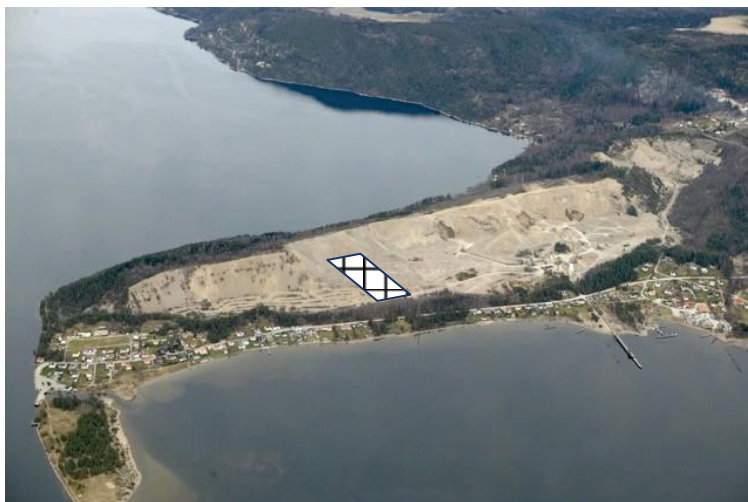
Fig. 1. Aerial photo looking northwards to the Svelvik ridge at the outlet of the Drammensfjord. The sill is formed by deglaciation deposits. The photo shows the sand excavation on the ridge. The laboratory location is indicated by the white rectangle (extension is approximately 300 m × 150 m).
