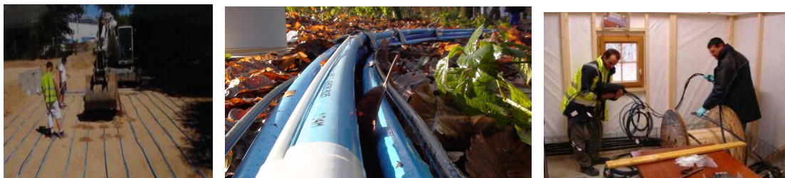
Figure 2. Deployment of one horizontal heat exchanger sector; HDPE pipe with its fiber along; fiber handling in the hut
