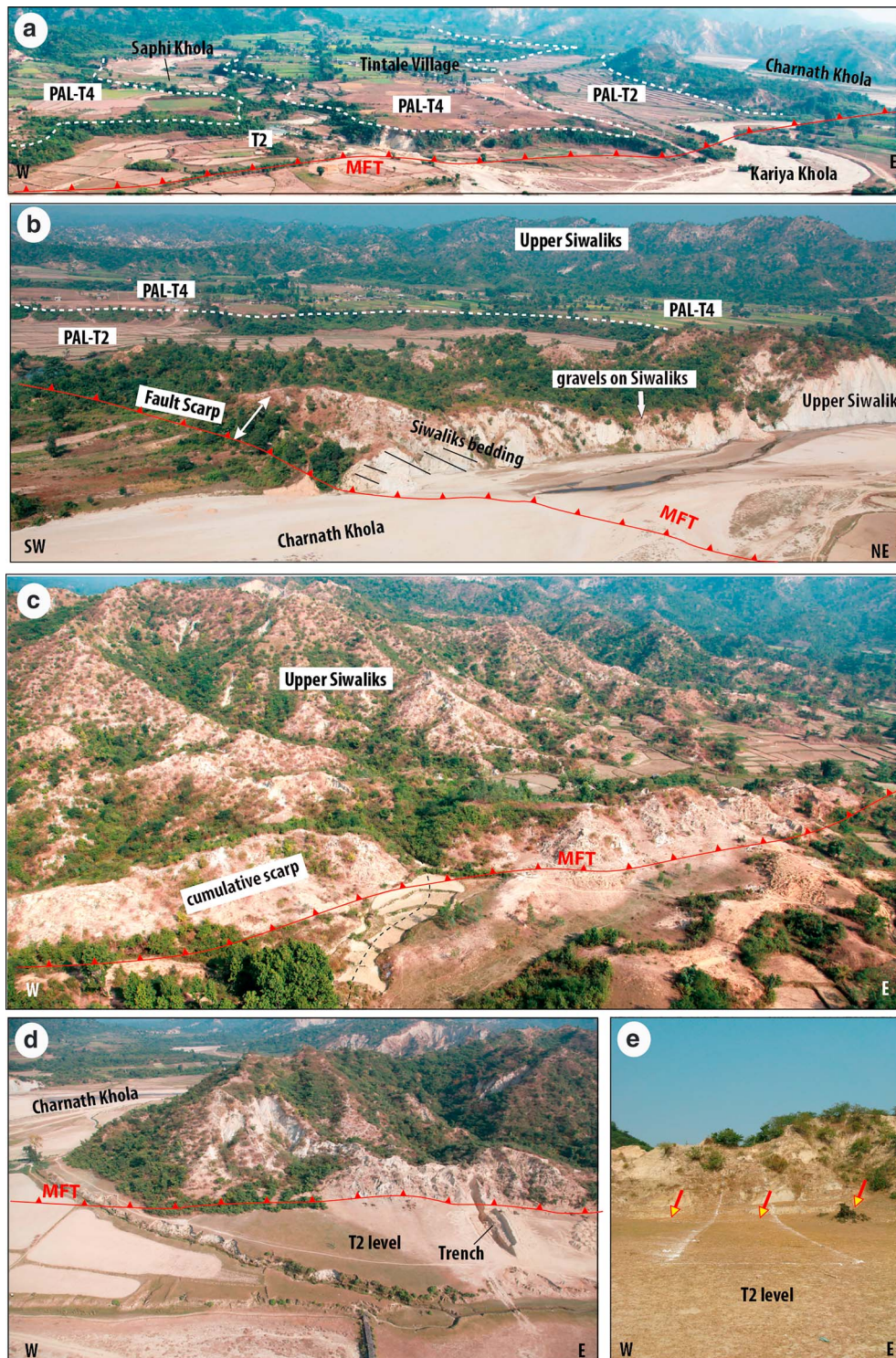
Figure 4. Helicopter views (taken on the 2nd of December 2009) of the cumulated fault scarp along the Charnath Khola MFT strand (see location in Figure 2). The red line represents the assumed trace of the MFT. (a) View on Paleomeander Pal-T4 and Pal-T2 at the confluence of the Saphi, Kariya and Charnath Khola (Tintale Creek). The white dashed lines highlight the alluvial levels. (b) The outlet of the Charnath Khola (river cut) where the MFT (in red) cuts the present-day riverbed. The white dashed line represents the top of the Pal-T4 level. (c) A 20- to 30-m high cumulative scarp east of the outlet of the Charnath Khola. (d) Helicopter view toward the north of the Front Range after the Cobra trench excavation. (e) Field view taken before the excavation. The red and yellow arrows locate the 1-m high scarp at the toe of the cumulative scarp. The white line on the photo delimits the location of the future trench.
