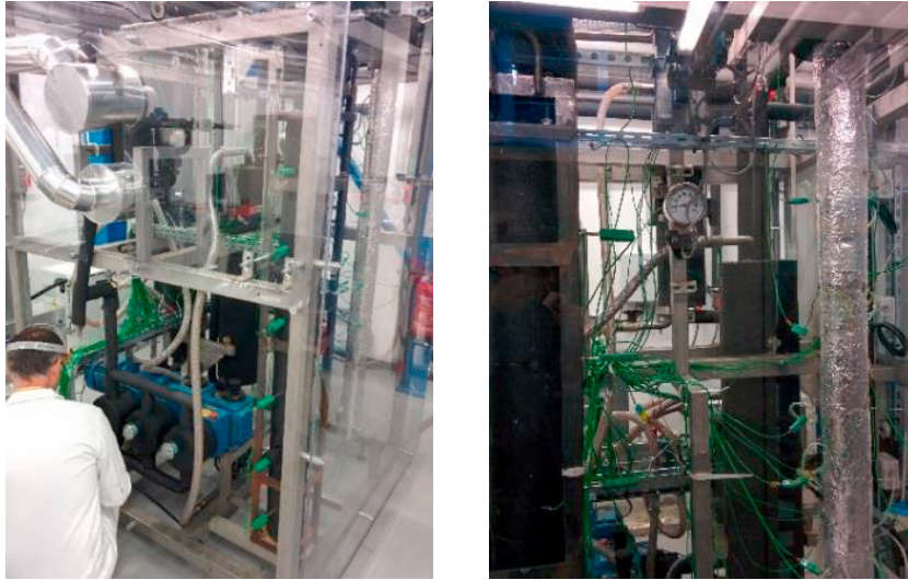
Figure 3. Photographs of CO2 loop and two vertical test sections
