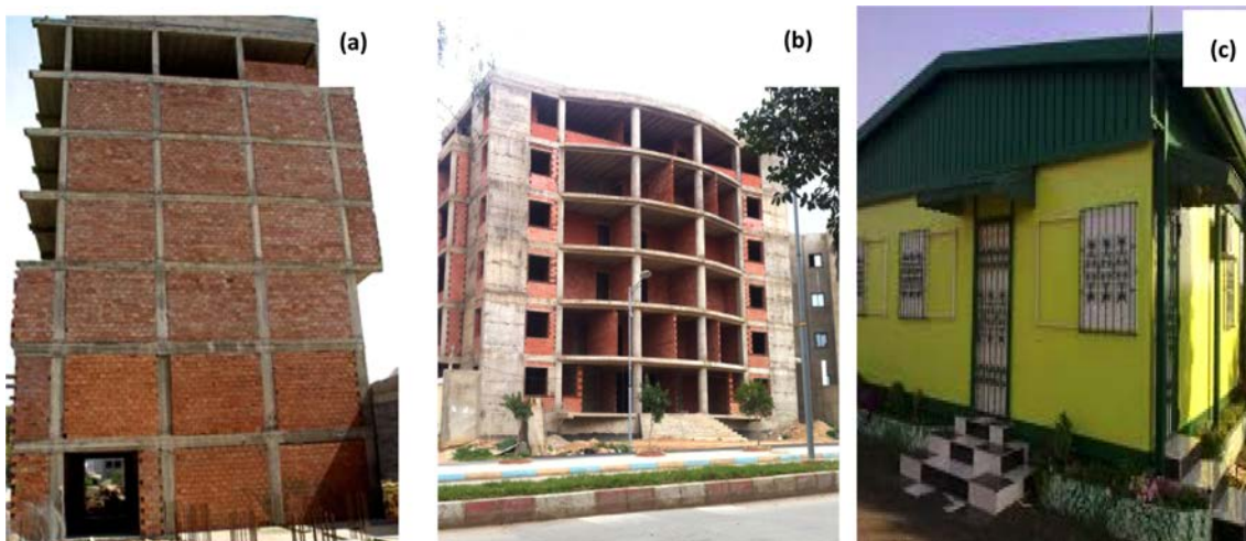
Fig. 3. The Main Building Typologies Existing in Chlef City Today: (a) RC Moment Frames (b), RC Shear Walls Buildings, (c) Prefabricated Houses
