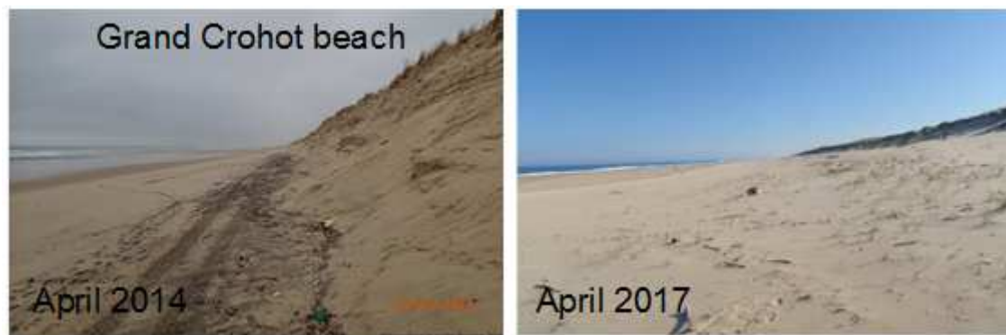
Figure 4: Photographs of the erosion dune scarp and foredune installation at the grand Crohot beach (Cell 3.4)
