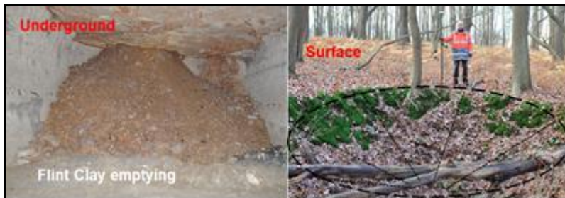
Figure 2. Example of an alteration root intercepted at the bottom, and of the fontis induced in the surface by its emptying
