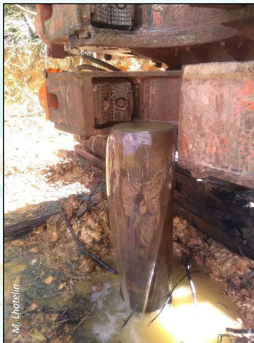
Artesianism on the PAP1 water well
