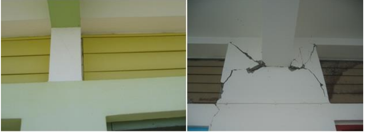
Figure 1: Diagonal cracks in the short columns
