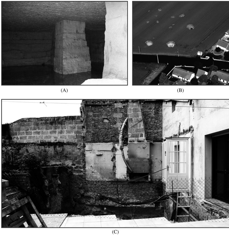
FIG. 1. (A) Building-stone underground quarry of Fleury-sur-Orne (Calvados, France) with pillars supporting the cavity roof, some reaching 10 m in height (© E. Plat – BRGM 2014). (B) Thirteen sinkholes formed following exceptional rainfall in late May 2016 in the village of Gidy, central France. These sinkholes turned out to be located above a forgotten quarry (© T. Dewez – BRGM 2016). (C) Damage caused by sinkhole collapse to a house in Doué-la-Fontaine (Maine-et-Loire, France). The extension to the main house entirely disappeared into the 400 m 3 sinkhole (© E. Plat – BRGM 2011).
