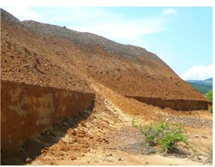
Tailings dam failure and tailings escaping towards the river
