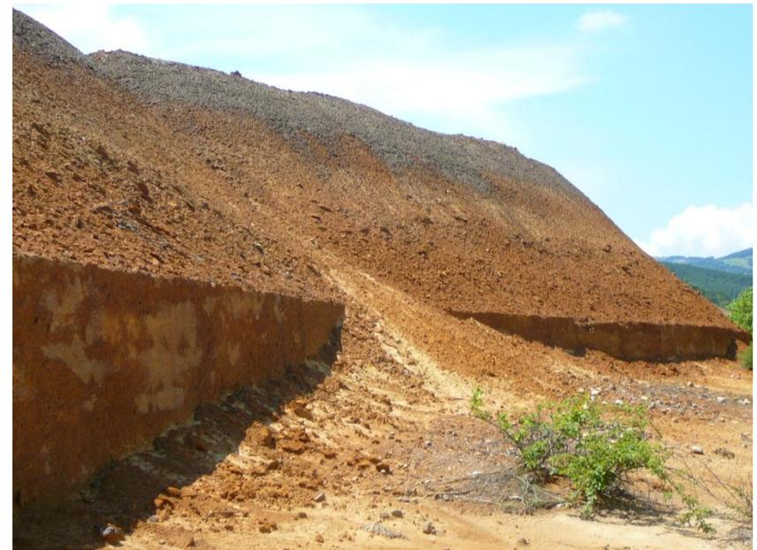
Tailings dam failure and tailings escaping towards the river
