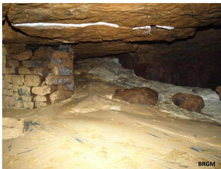
Figure 8: injection into the cavity in Franchepré in Moyeuvre-Grande (57)
