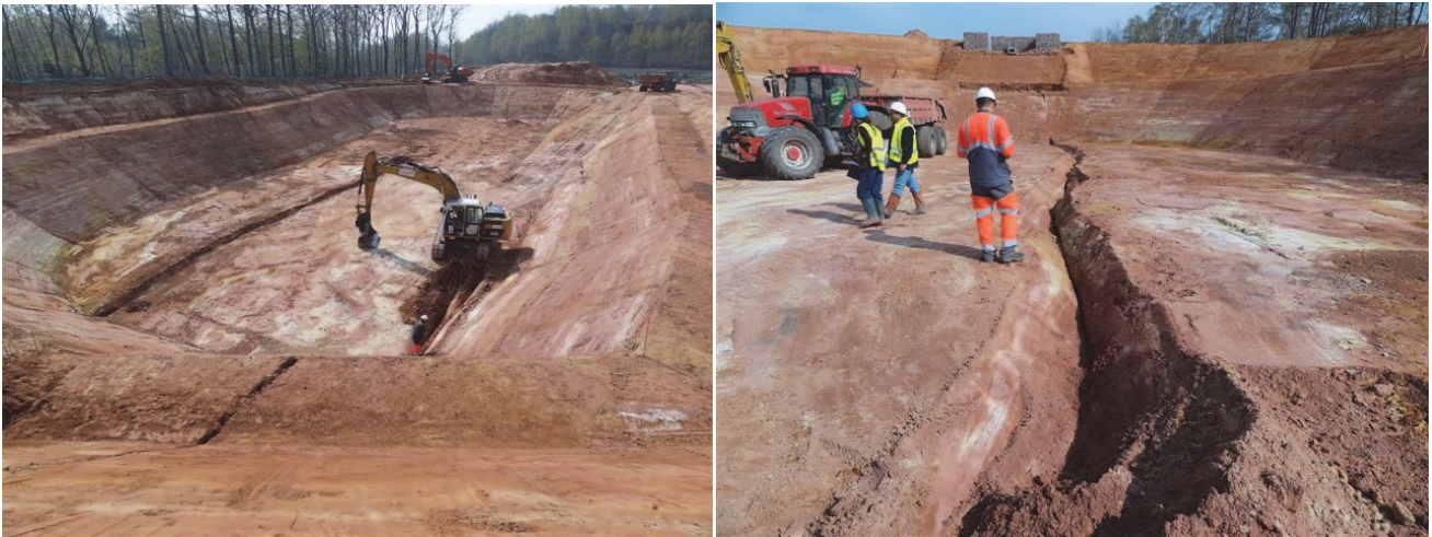
Figure 6. Terrassement des crevasses – Bassin 2 – 05/04/12
