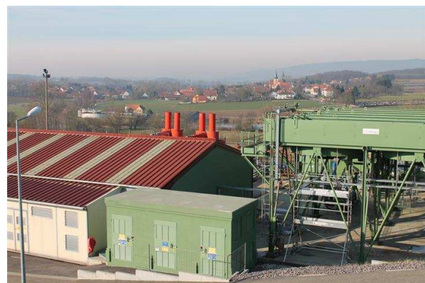
Figure 1: The Soultz power plant with the village of Kutzenhausen in the back.
