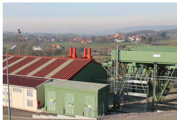
Figure 1: The Soultz power plant with the village of Kutzenhausen in the back.
