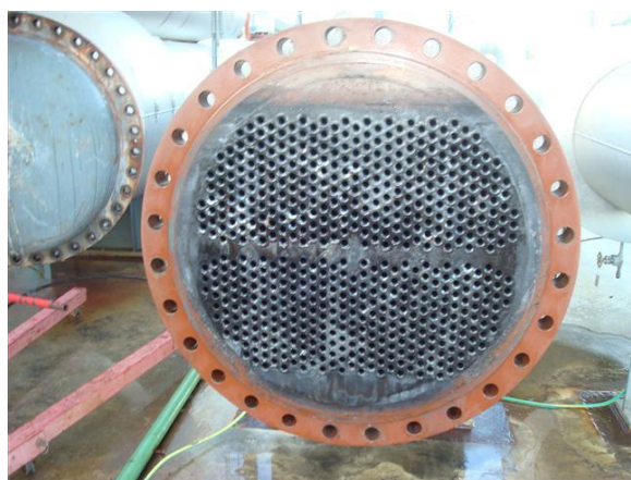
Figure 10: Black scaling observed within the heat exchanger during exploitation.
