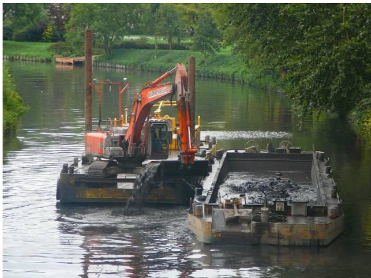
Figure 2. Bulk dredging, Lens canal, 2010
