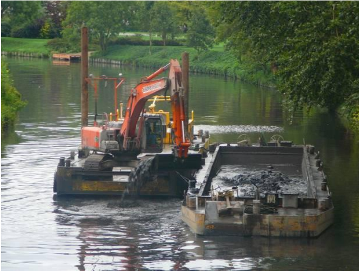
Figure 2. Bulk dredging, Lens canal, 2010
