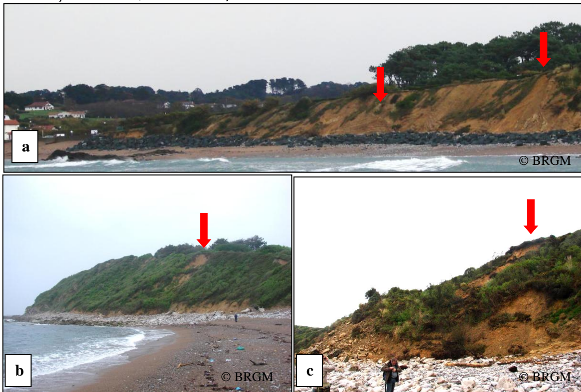
Figure 6 Different instability areas on Erromardie beach. The red arrows point at recent landslides.
