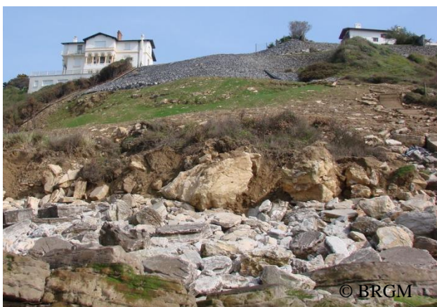
Figure 8 Construction of a draining blanket over slid materials.
