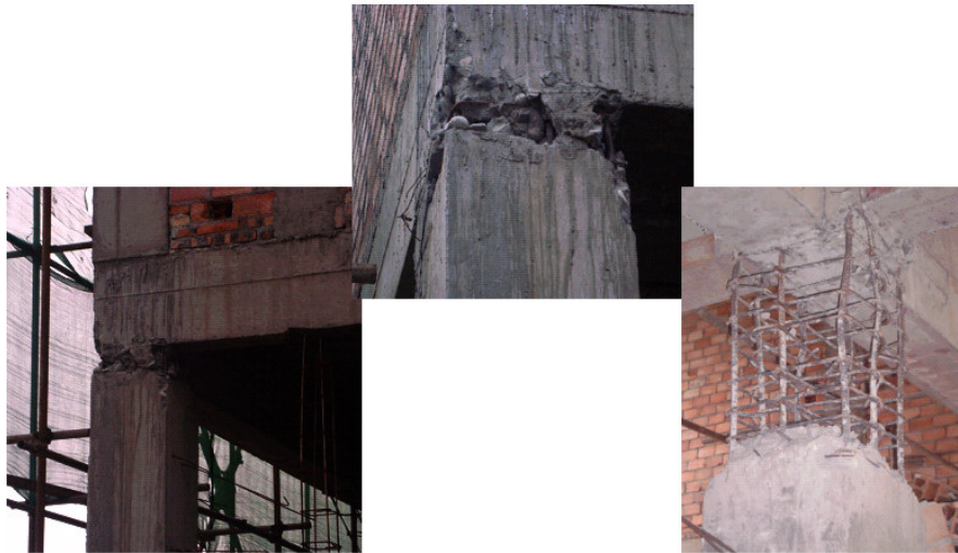
Figure 2 – Examples of damage to RC frame buildings. Photographs taken by S. Ghavamian in Dujiangyan following the 2008 Sichuan earthquake
