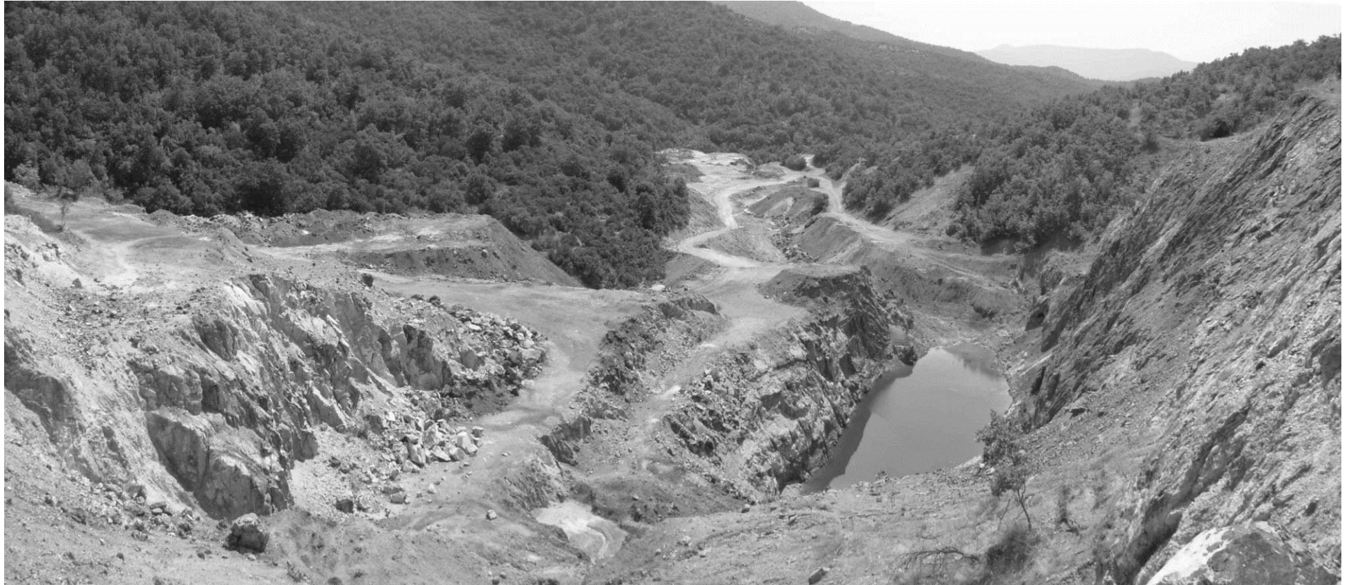
Figure 4. General view of the open pit mine area. Mining waste dumped downstream and waste heap drainage escaping towards the brook.
