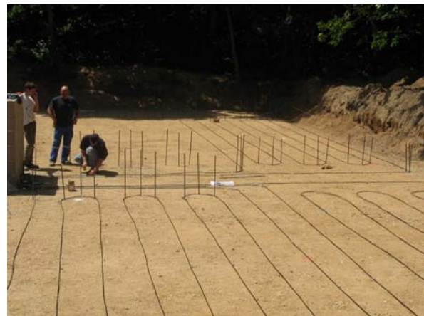
Figure 7: Implementation of the optical fibers at 1.5 m
