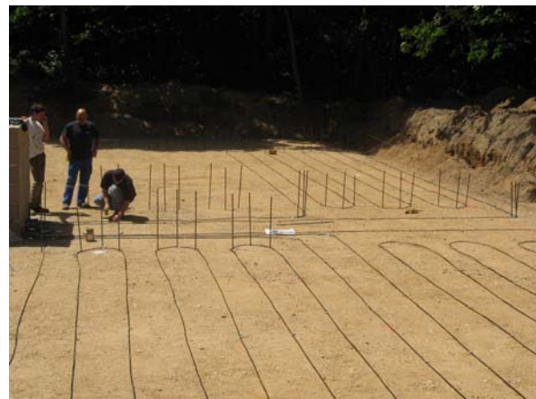
Figure 7: Implementation of the optical fibers at 1.5 m
